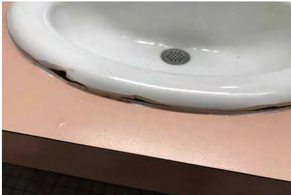
#33 DAMAGED SINK
