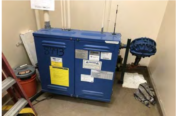
#28 HYDRAULIC ELEVATOR
