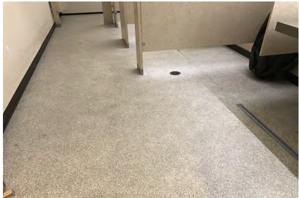
#16 RESTROOM VINYL FLOORING
